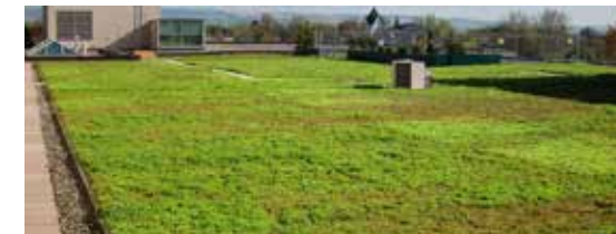
6 Green Roof Planting - Sedum Mix
