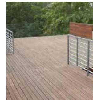
3 Wood Decking on Pedestal System
