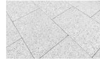
1 2' x 2' Precast Concrete Pedestal Pavers
